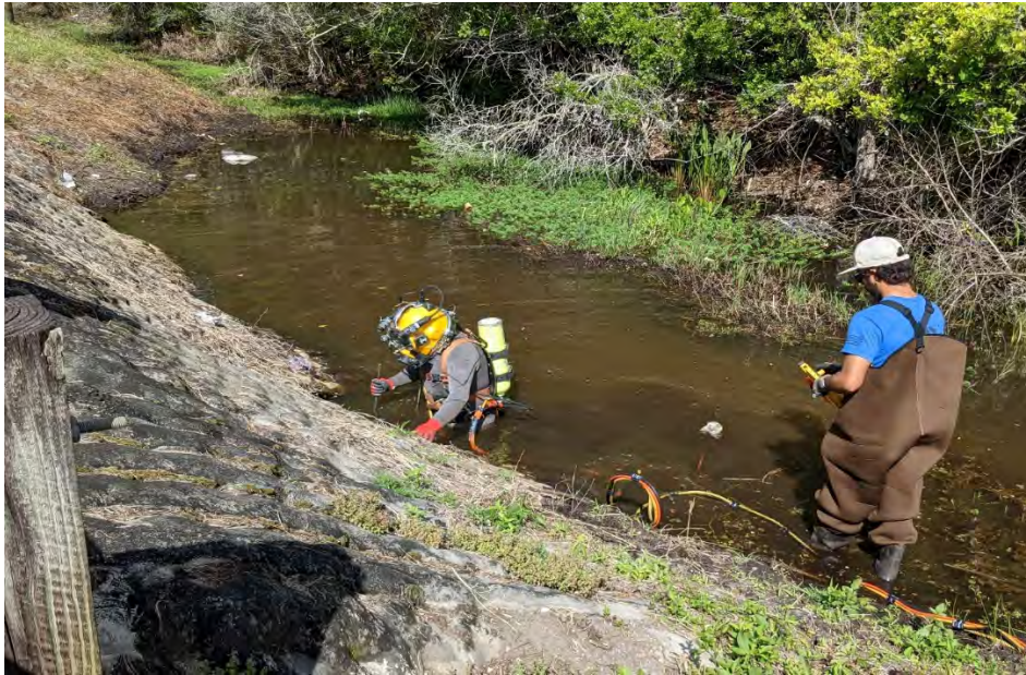
Pipe Inspections of Major Pipe Crossings
