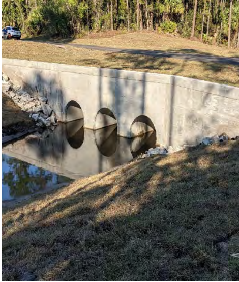
K-6 Weir Replacement- Complete
