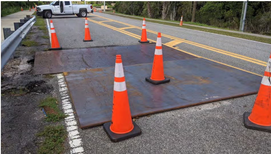
K-9 Emergency Pipe Replacement –Before Construction
