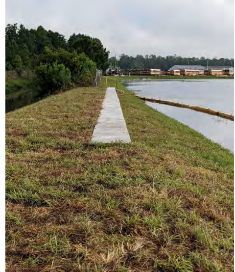
FPC Berm Rehabilitation – Complete
