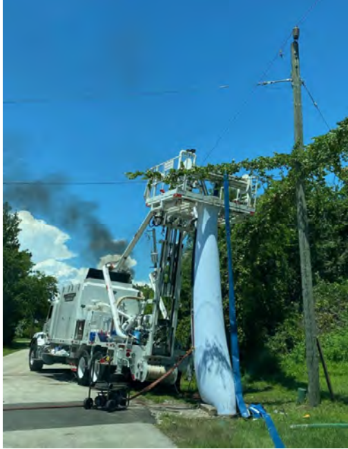
Cured in Place Pipe (CIPP) Lining – Persimmon Drive
