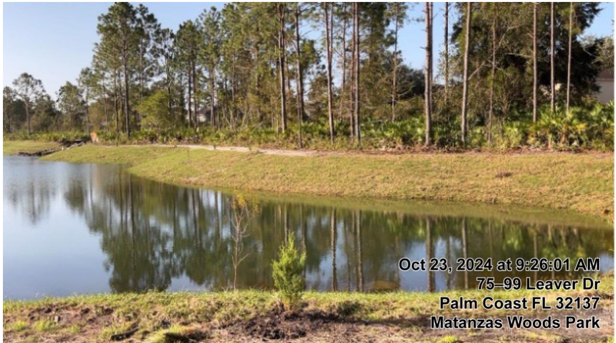
Figure 2: London Waterway finished construction
