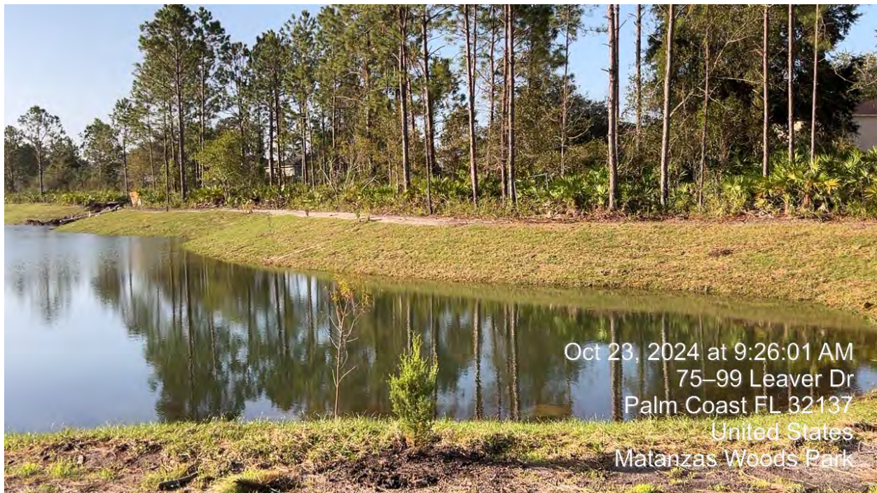
Figure 1: London Waterway finished construction
